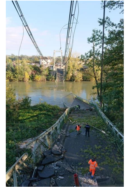
Collapse of the Mirepoix, France, suspension bridge because of an overloaded truck (2019)
