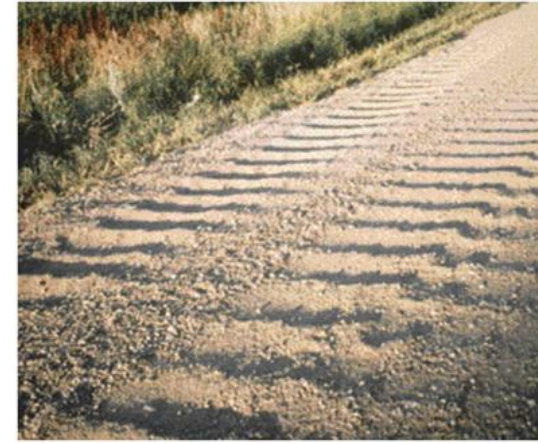
Distresses of unbound pavements: corrugation (Skorseth & Selim, 2000)
